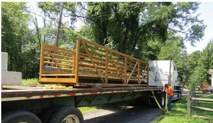
Footbridge arrives at W. Watson Avenue park entrance.
