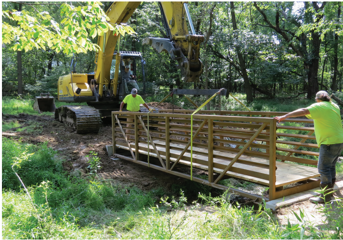
Footbridge is placed on concrete footers.
