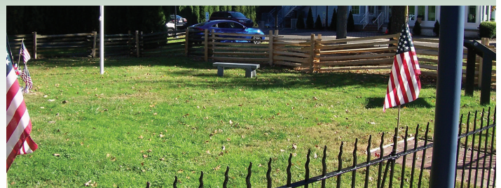
Foreground: Newly painted wrought iron fence; Background: Restored colonial era fence.
