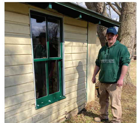
Chris Fullan after reinstalling the windows.
